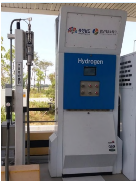
Hydrogen dispenser in South Korea using IRDI System parts supplied through its German partner, WEH. (Source: IRDI System)
