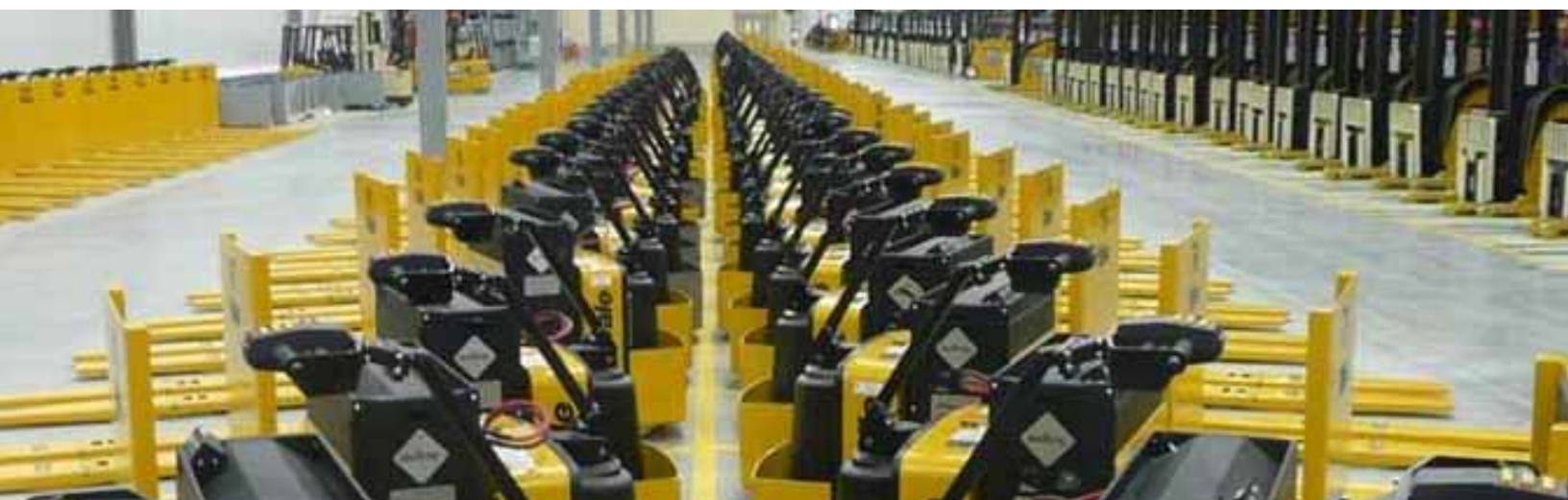
The entire fleet of material handling equipment at the new Walmart Perishable Distribution Centre in Balzac Alberta is powered by hydrogen fuel cells
