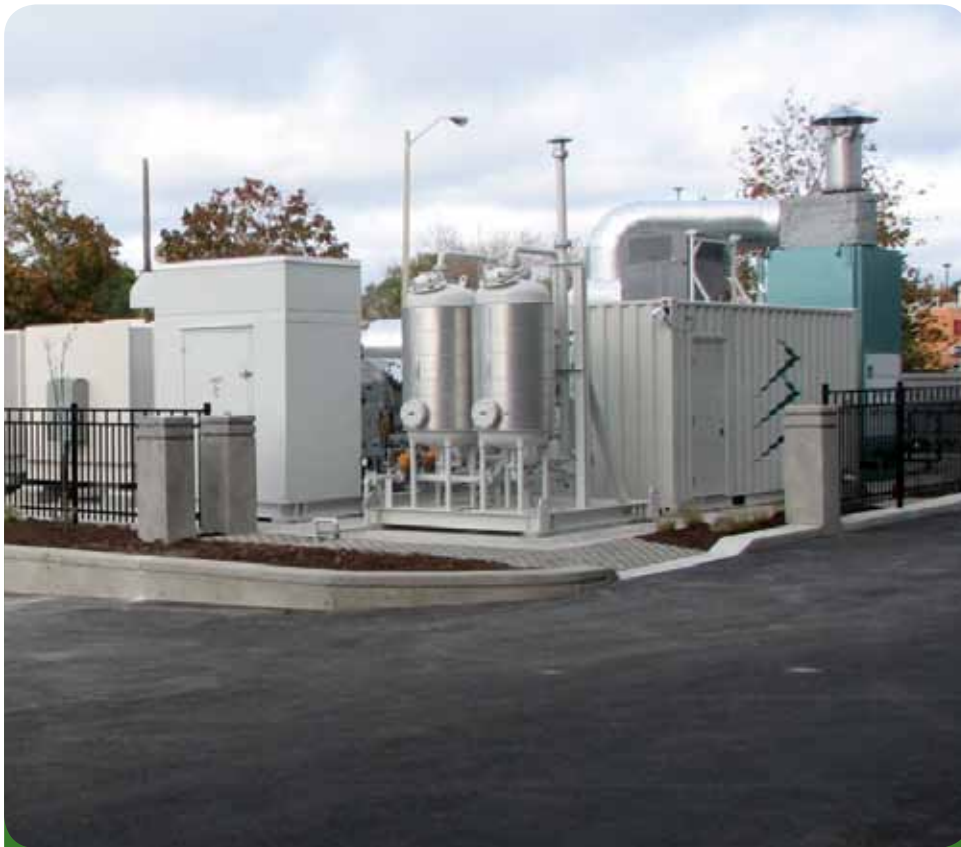
Photo: Enbridge Gas Distribution and Fuel Cell Energy | Direct Fuel Cell-Energy Recover Generation Power Plant in Toronto, Ontario
